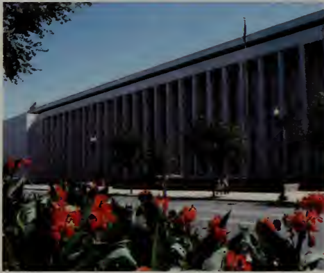
James Madison Memorial Building.
